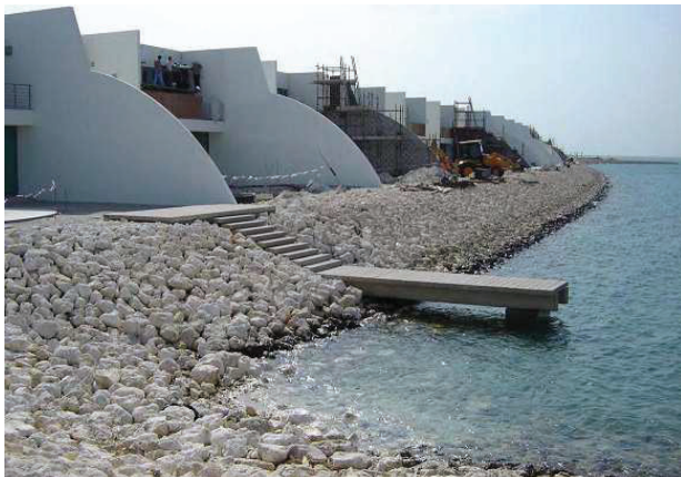
PermaTrak Sundeck, Steps and Pier - Bahrain
