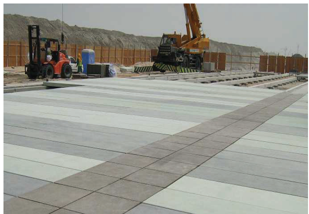
PermaTrak promenade construction – Palm Deira
