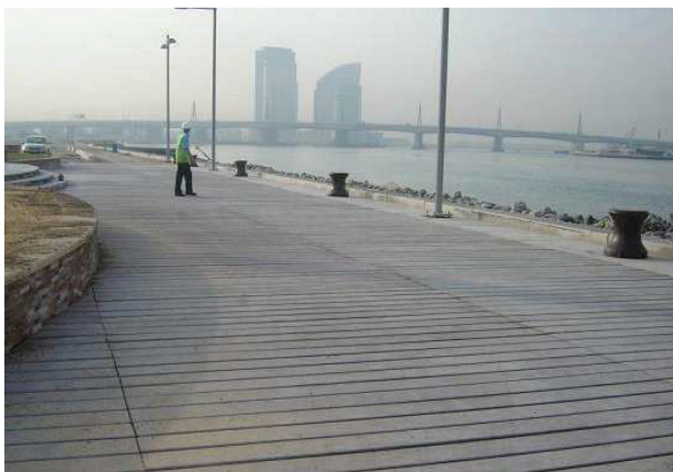
PermaTrak Promenade Deck - Dubai Corniche
