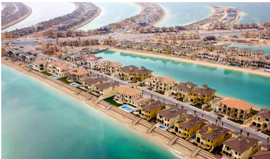
Sea shore retaining walls for Palm Jumeirah
