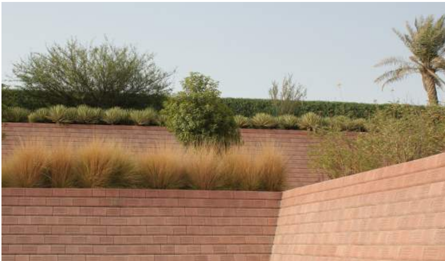
Double layer terracing, sloped wall
