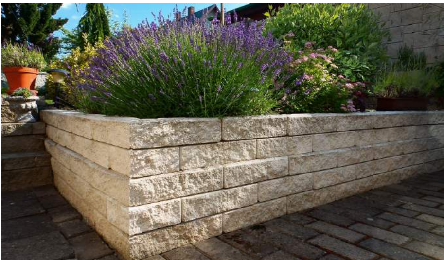
Stavoblocks used as a raised planter bed
