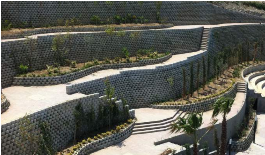
Retaining wall with pedestrian access
