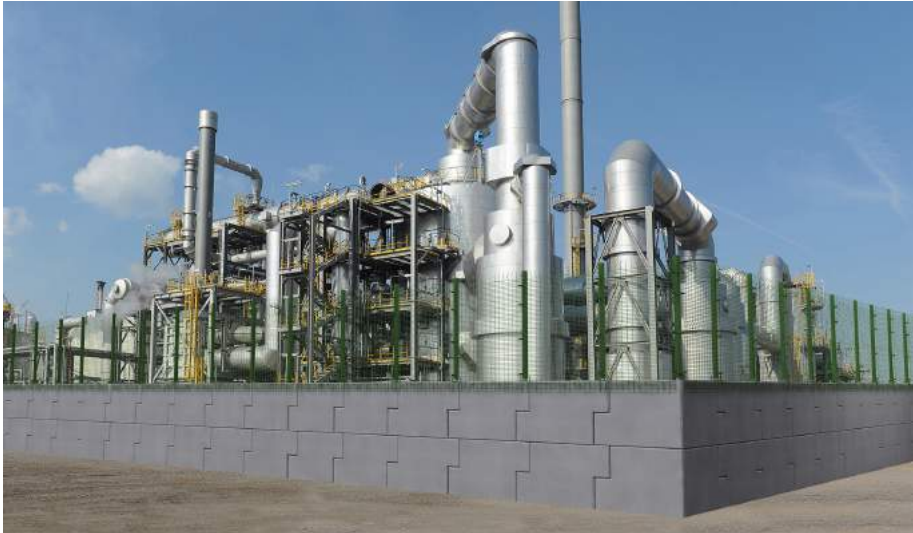
Double layered with fencing installed on top for extra security
