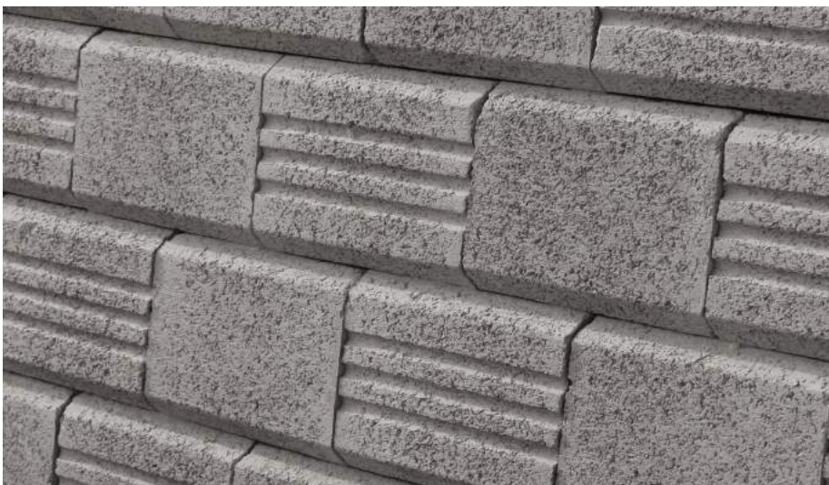
Close-up of blocks
